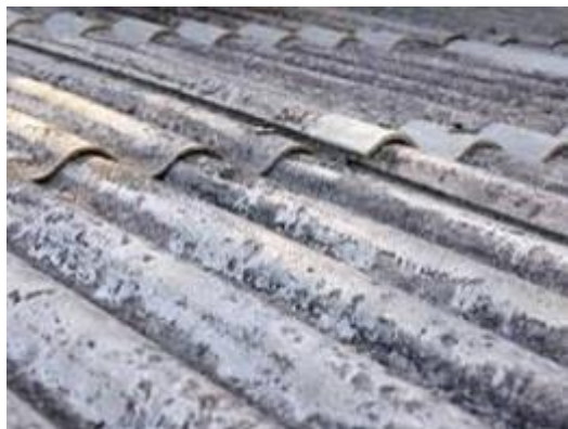
Asbestos panelling
